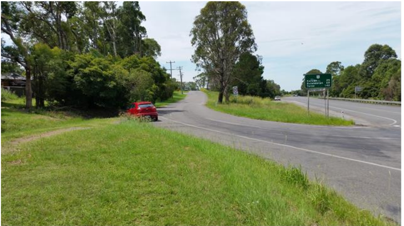
Photo 6: Rees James Road (Approx. Chainage 2200 looking North – Eastern Route)
