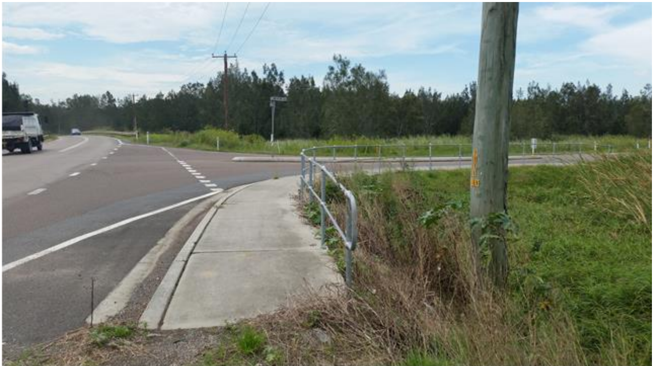
Photo 10: Cnr of Newline Road and Beaton Avenue (Approx. Chainage 2400 – Western alignment)
