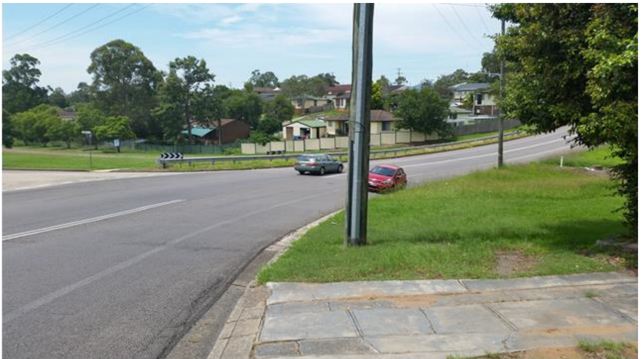
Photo 2: Mount Hall Road (Approx. Chainage 800 looking North)
